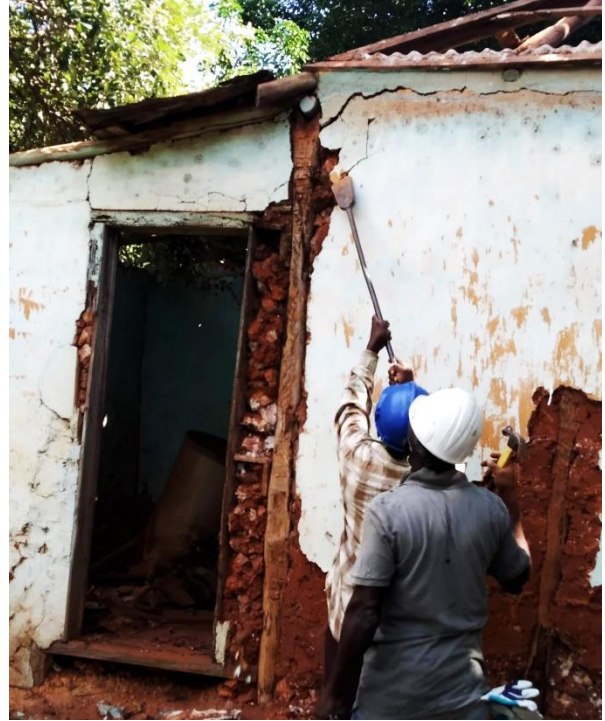
“Testing the Structure” (© Carol Campbell, January 2021)
