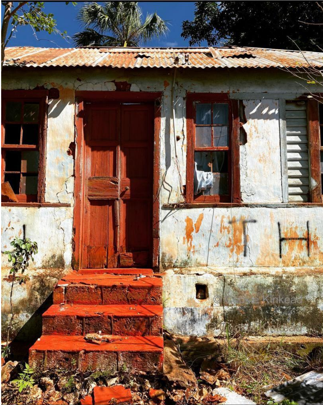
The Vassel House - South wall (© Cookie Kinkead, January 2021)
