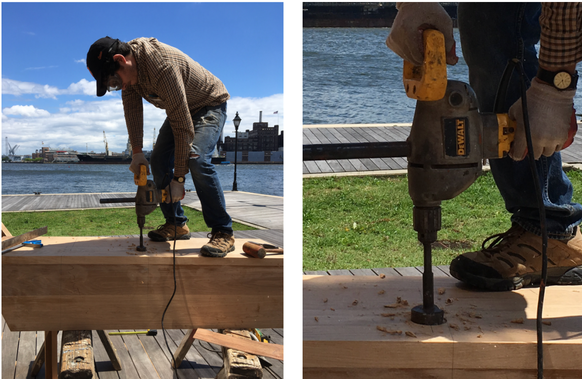
Figure 2: The author drilling holes in a cat-head (left); close-up of the tool with Forstner bit attached (right)
