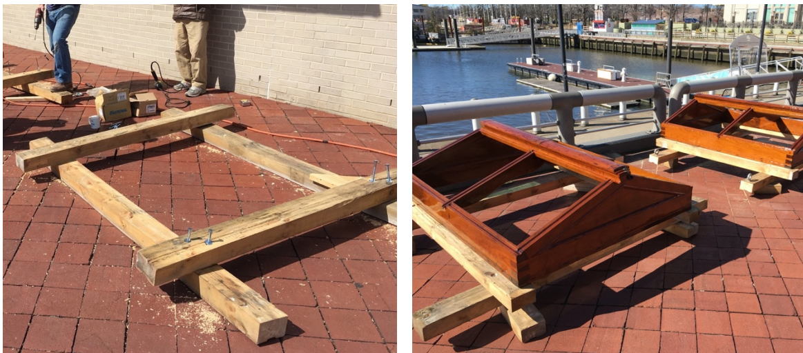
Figure 1: The cradles under construction (left), and the cradles in use (right)
